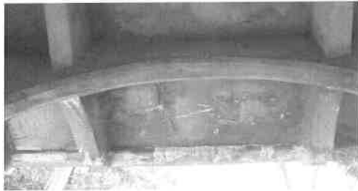
1935 sidewalk /railing replacement
